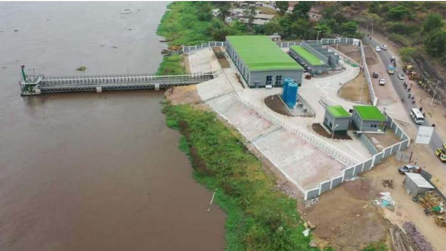
Station de captage Ozone
