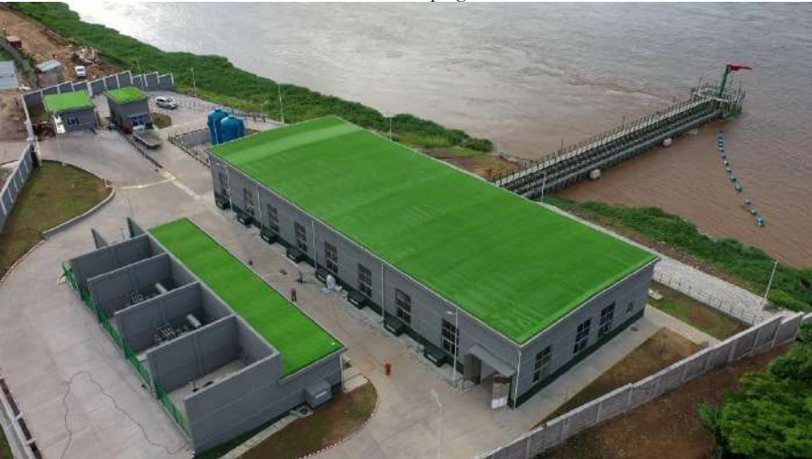
Station de captage Ozone
