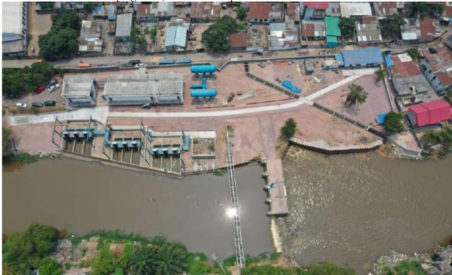
Station de captage N'djili
