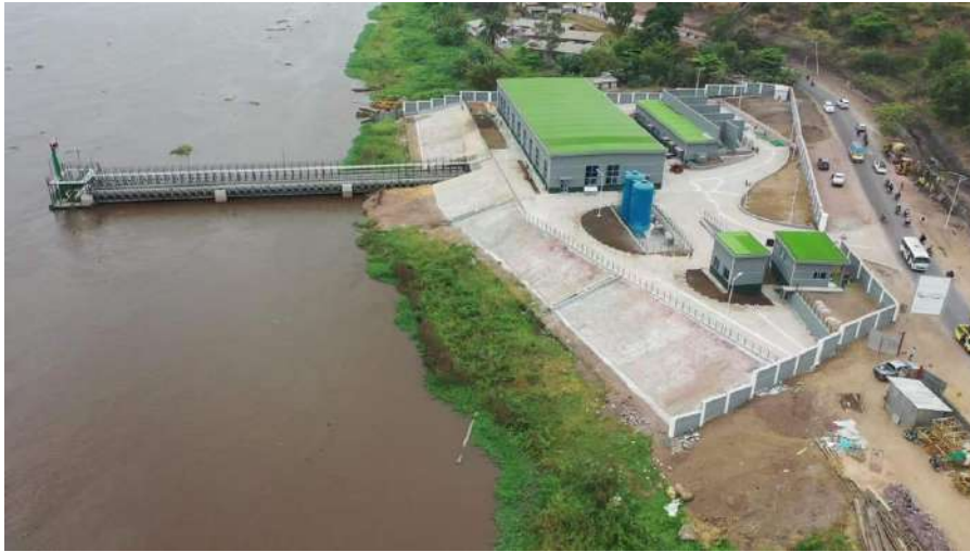
Station de captage Ozone
