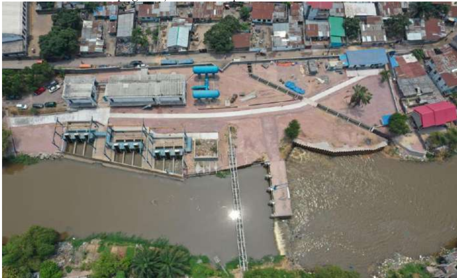
Station de captage N'djili
