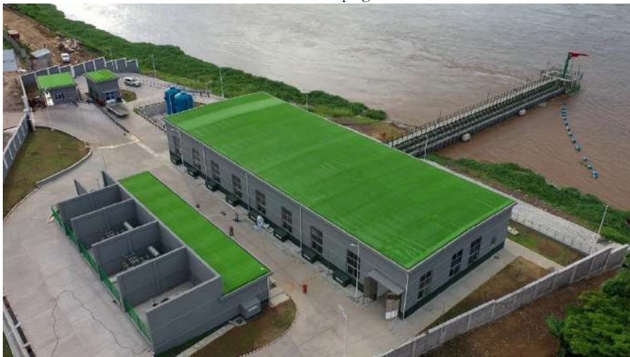
Station de captage Ozone
